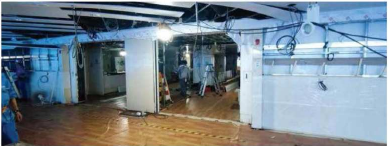
Electric Sliding Door (A60)
